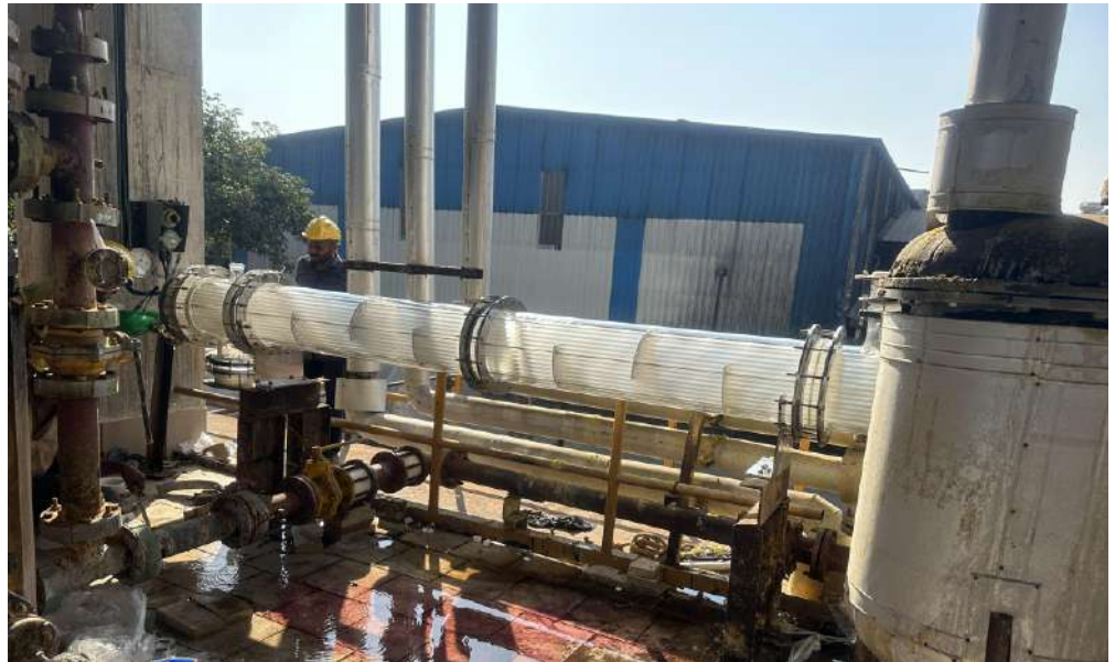
Borosilicate glass 3.3 Shell and Tube Heat Exchanger
