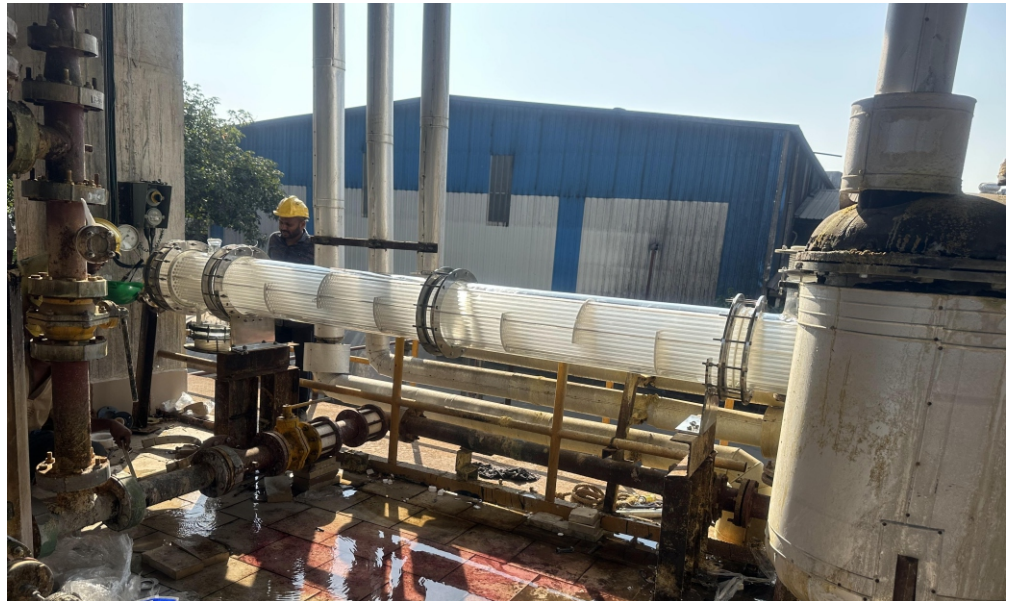
Borosilicate glass 3.3 Shell and Tube Heat Exchanger
