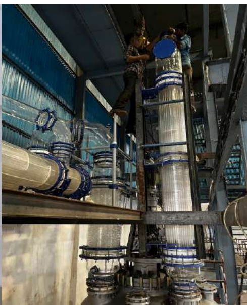
GLR Overhead Borosilicate Glass 3.3 Assembly
