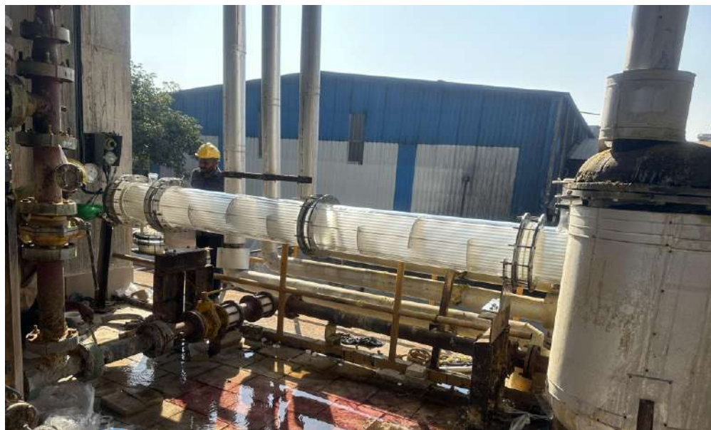
Borosilicate glass 3.3 Shell and Tube Heat Exchanger
